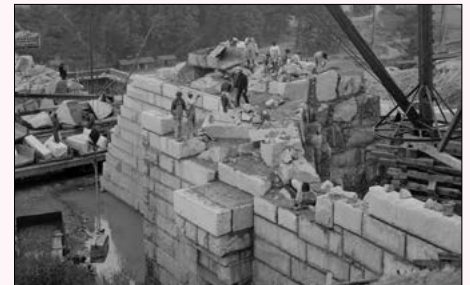
Building the Wachusett Dam.
